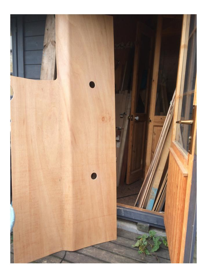
I opted for invisible fixings called "Big Hat Poppets" These are a two part push fit, one glued to the substrate to be held up the other to the ceiling so they are all glued in place after only needing to scrape a small area for the epoxy to bond. They are then clipped together and the covered in epoxy and the substrate pushed up against the plastic part of the poppet.
